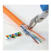
2. Fan out all 4 twisted pairs, allocate each conductor into the proper slot on the wiring cap by following the colour coding label. Trim the excess lenghts.
